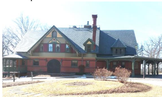
Carriage House from the estate that became Forest Park
